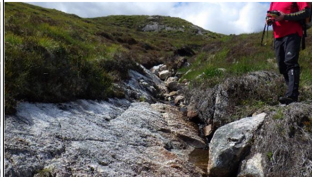
View upstream (west) at NH 3639 6689 showing incised bedrock channel with unstable banks and substantial rocky debris.
